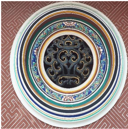
Figure 5: Brick Carving and Brick Laying
